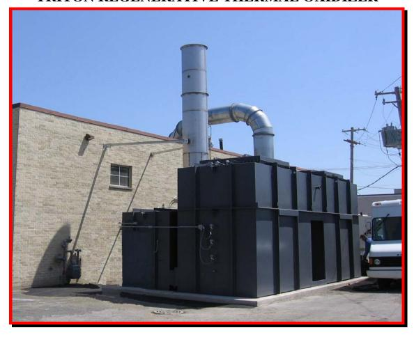
A heat-set/web offset printer recently installed a TRITON-Regenerative Thermal Oxidizer from Catalytic Products International, Inc. The TRITON system was contracted on a turnkey basis, in which CPI engineered and installed; the ductwork system from all dryers, foundation work, electrical integration, and rigged the oxidizer. The project was installed on time and without any added costs.
