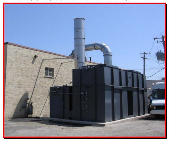
A flexographic printer recently installed a TRITON-Regenerative Thermal Oxidizer from Catalytic Products International, Inc. The TRITON system was contracted on a turnkey basis, in which CPI engineered and installed; the fugitive enclosure system to meet method 204, the ductwork system from all presses, foundation work, electrical integration, and rigged the oxidizer. The project was installed on time and without any added costs.
