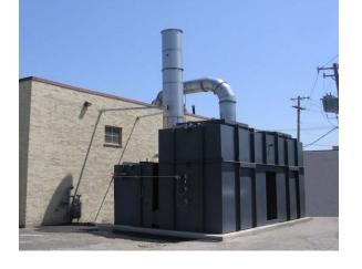
Permanent Total Enclosure or PTE is a method of collecting fugitive emissions from sources that do not have ducted exhaust points. The benefit of using a PTE is realized in many operations because:
