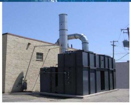
A surface coater recently installed a TRITON-Regenerative Thermal Oxidizer from Catalytic Products International, Inc. The TRITON system was contracted on a turnkey basis, in which CPI engineered and installed; the fugitive enclosure system to meet method 204, the ductwork system from all presses, foundation work, electrical integration, and rigged the oxidizer. The project was installed on time and without any added costs.
