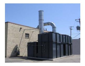
Permanent Total Enclosure or PTE is a method of collecting fugitive emissions from sources that do not have ducted exhaust points. The benefit of using a PTE is realized in many operations because:
